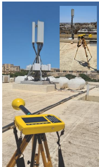
Figure 4: In-Situ EMF Measurement Site #2 (co-hosted)
