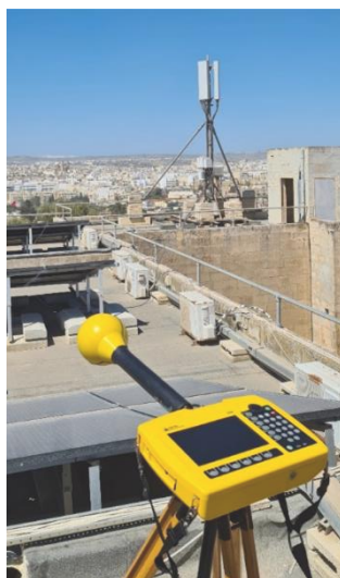
Figure 3: In-Situ EMF Measurement Site #1
